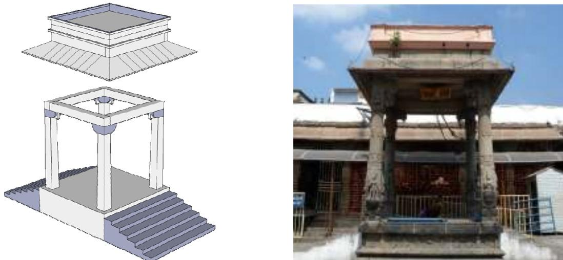
**Fig. 1** Schematic representation of the 4-pillars mandapam, with clear distinction between the resisting and the roofing systems (left) and front view of the real structure at Triplicane, Chennai, India (right).
